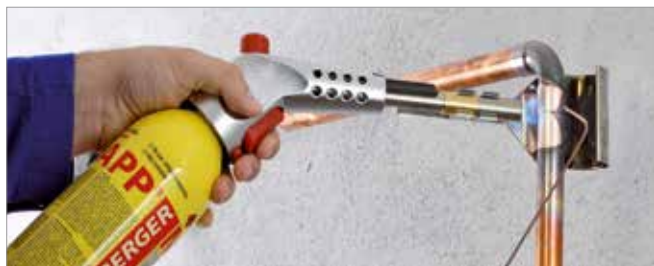
Brazing in gas installation
