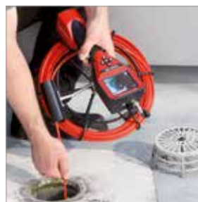
Inspection of rain downpipes
